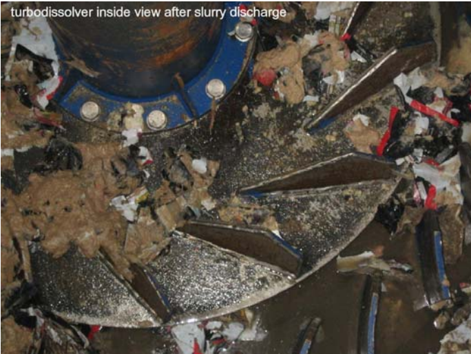
turbodissolver inside view after slurry discharge
