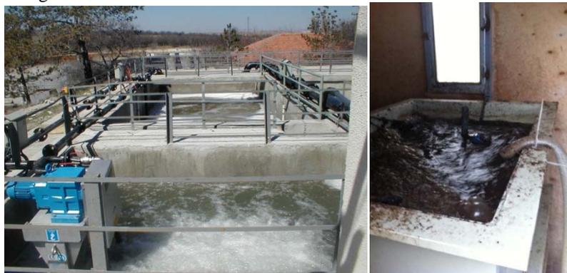
**Figure 1** Pictures of the full-scale VRM (left) and pilot scale MBR units at METU Campus, Turkey.
